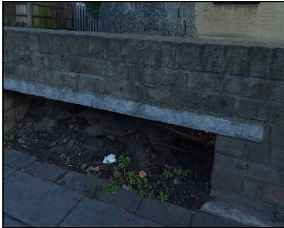
Photograph 4 – Example of wall bridge over tree roots
